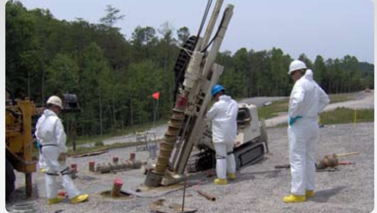
Collar pipe installation at ORNL trench.
