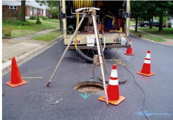
Figure 3: Grout Rig
